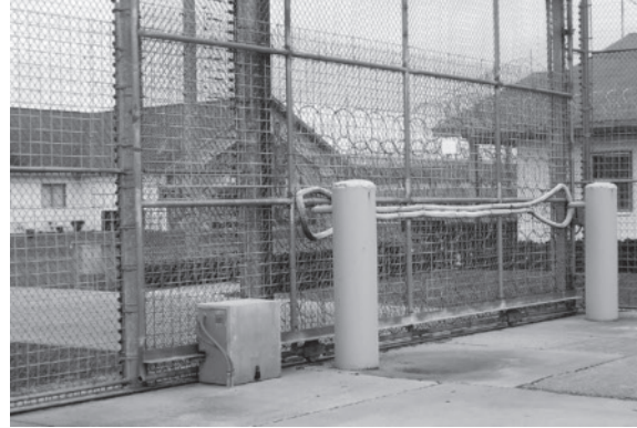
Figure 4-4 An exterior sally port gate large enough for vehicles to pass through
