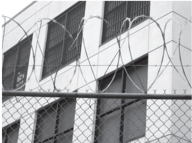
Figure 4-5 Razor wire tops a fence on the perimeter of a correctional facility
