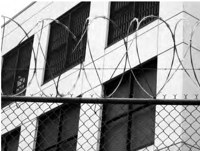
Figure 4-5: Razor wire tops a fence on the perimeter of a correctional facility
