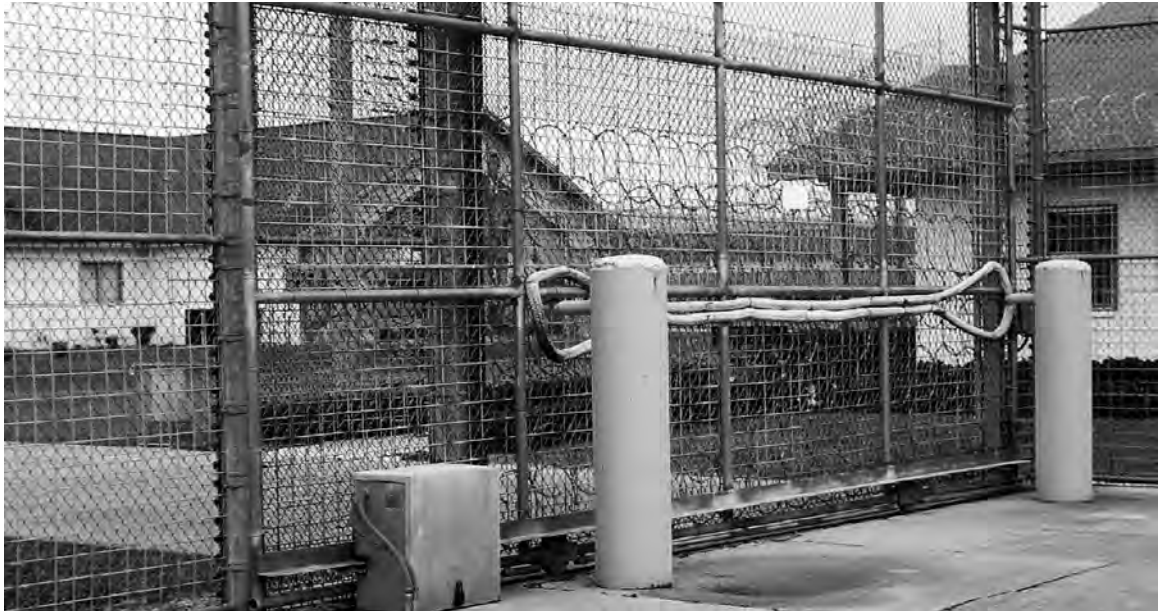
Figure 4-4: An exterior sally port gate large enough for vehicles to pass through
