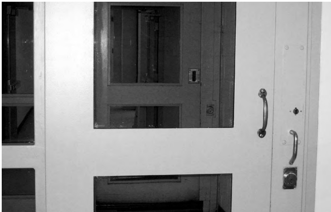
Figure 4-1: Doors that allow one section of passage to be closed before opening another section
